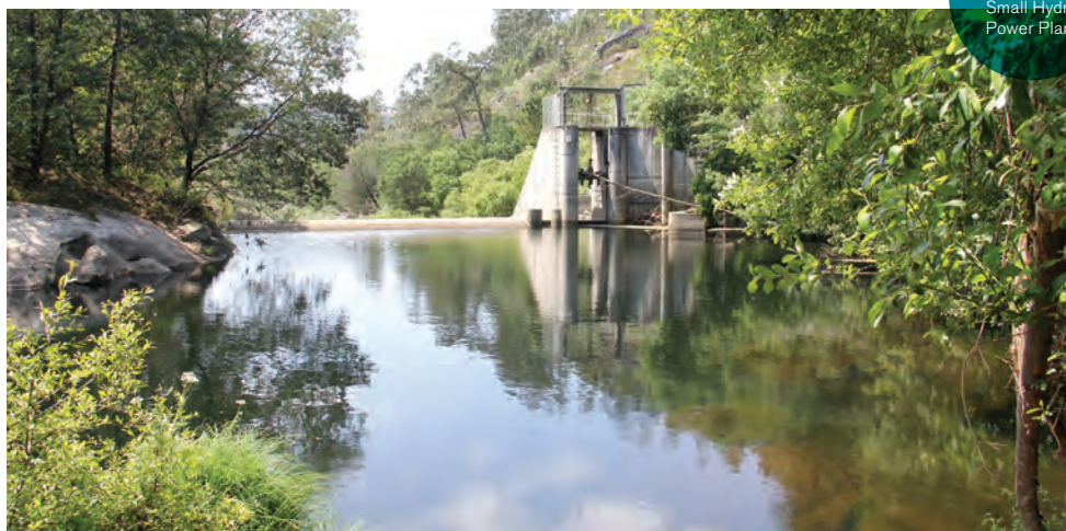
TALHADAS Mini-hídrica Small Hydro Power Plant
