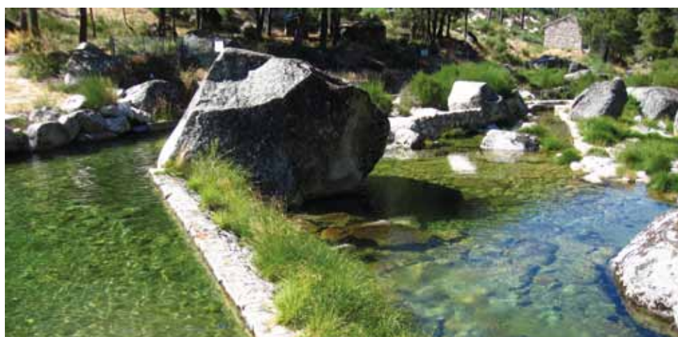
MANTEIGAS Mini-hídrica Small Hydro Power Plant
